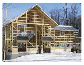
Figure 5. Project 1: Wall framing during construction
