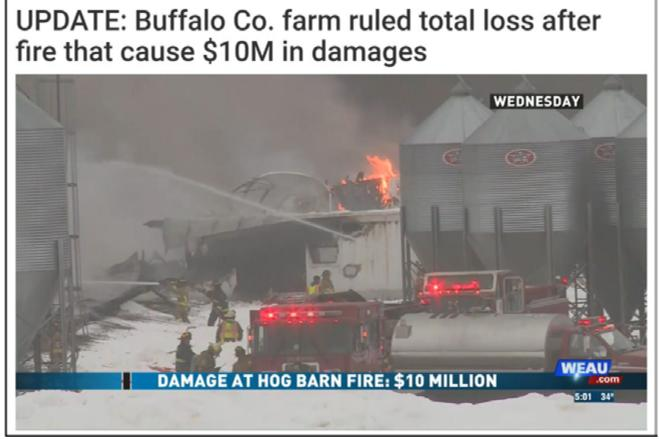
Figure 5: A post-frame hog barn collapsed in Wisconsin after a March 2019 snow event which then caught on fire from an electrical source. The building was engineered for a 30psf Roof Snow load, less than the ASCE 7 standard for the building's location.
