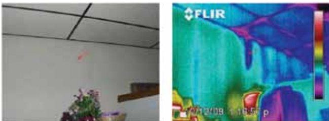
Figure 14. Air infiltration into a wall cavity during blower door testing.
