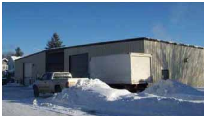
Figure 6. Rear view of low-rise steel-frame building involved in thermal envelope study.
