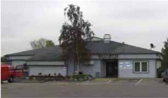
Figure 13. Wood stud-framed building involved in thermal envelope study.
