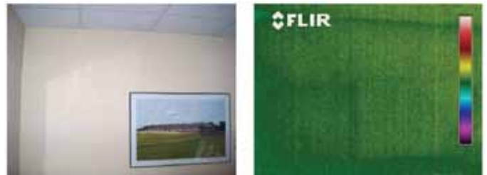
Figure 4. Typical exterior wall. Thermogram indicates no abnormal heat transfer.
