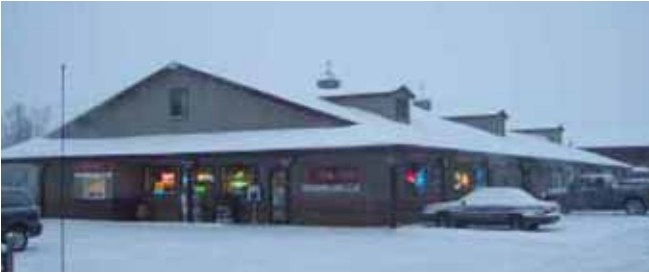
Figure 2. Post-frame building involved in thermal envelope study.
