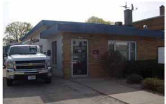
Figure 11. Masonry building involved in thermal envelope study.
