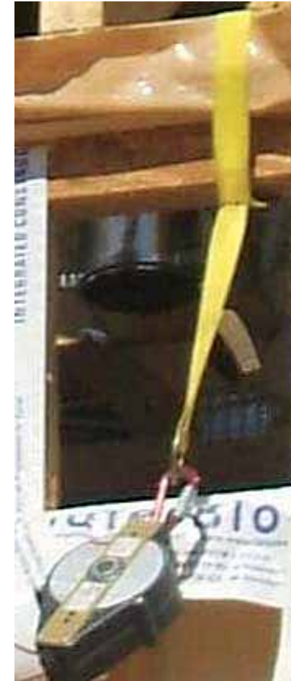
Figure 1 Photo from OSHA 2011 guidance document showing a questionable attachment to a wood member.
