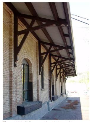
Figure 1-74. Wall support brackets used to support an eyebrow overhang.
