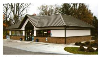
Figure 1-34. Small commercial post-frame building sided with stucco and brick veneer.
