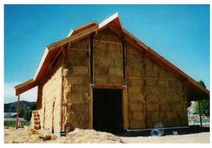
Figure 1-56. Non-structural straw bale walls prior to plastering. Image from the American Society of Agricultural and Biological Engineers. Used with permission.
