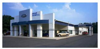
Figure 1-36. Commercial post-frame building clad in stone and smooth metal panels. An FBi Buildings project.
