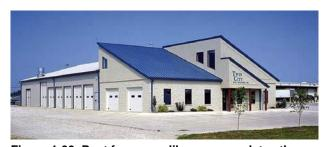
Figure 1-39. Post frame readily accommodates the overhead doors required for this automobile repair business in Lafayette, Indiana. An FBi Buildings project.
