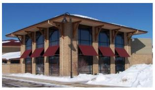
Figure 1-76. Tall walls, large regularly-spaced windows and wall brackets make buildings similar to this good candidates for post-frame.
