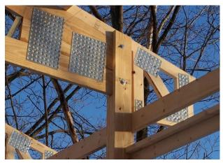
Figure 1-55. When truss is sandwiched between outer plies of a mechlam post, bolts are placed in double-shear for a very effective connection.
