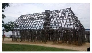
Figure 1-28. Frame of pole building barrack erected in 2011 in an effort to duplicate construction methods used during the colonization of Jamestown. Located behind the replicate barrack is a replicate palisade.
