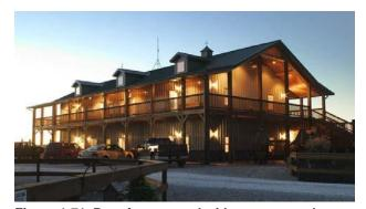
Figure 1-71. Post-frame motel with wrap-around balcony.
