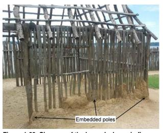
Figure 1-29. Close-up of the barrack shown in figure 1-28. Embedded poles support a girder which in turn supports rafters. Note the similarities between this construction and that shown in figure 1-3.
