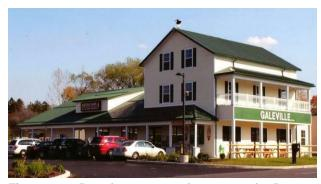
Figure 1-66. Post-frame convenience store for Byrne Dairy in Galeville, NY. The storefront features a porch and above balcony. A porch formed by a roof overhang extends along the side of the structure.
