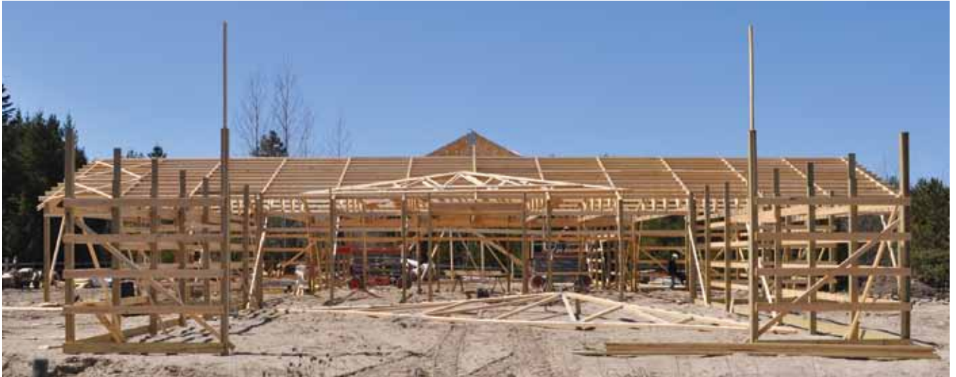
Figure 1. Splash plank and mechanically laminated posts. (Photo courtesy of Wick Buildings.)
