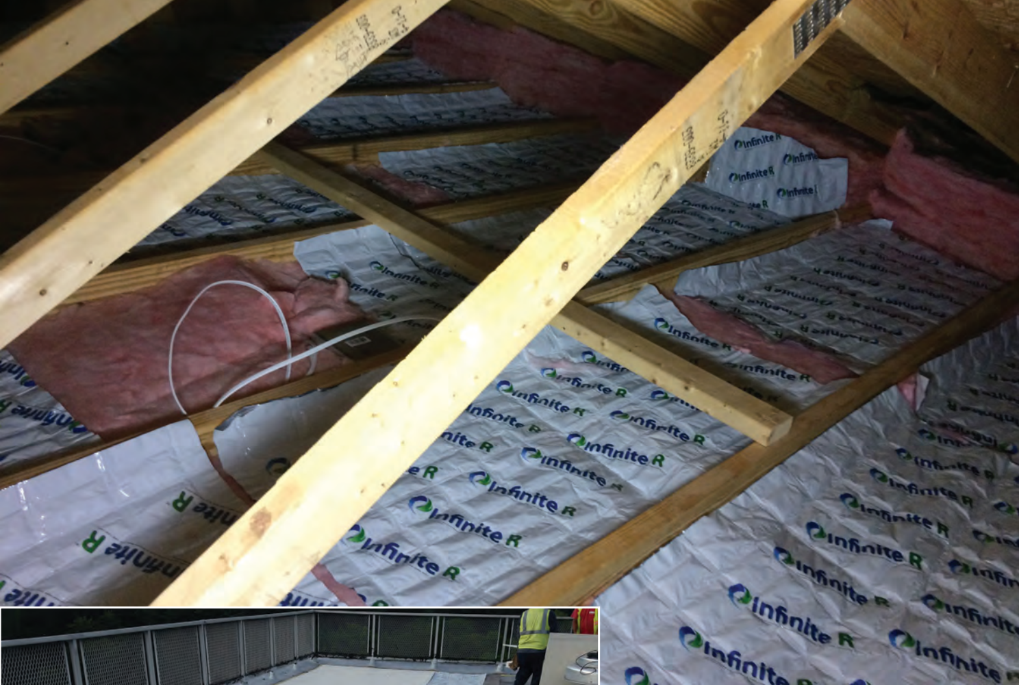
Figures 6 and 7. Phase-change materials can be used in the retrofitting of existing construction. Photos: Insulcorp.
