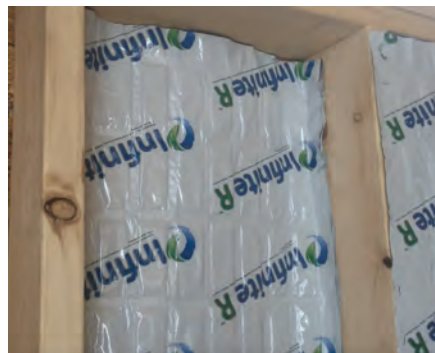
Figure 4. Pouches containing phase-change material are often attached to the inside of wall cavities, stapled to the inside of the sheathing or girts. Photo: Insulcorp.
