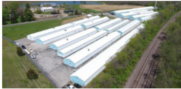
MiniMax mini storage complex where Matt has built almost 20 buildings for this customer between the complex shown, and the owners other mini storage complex.
